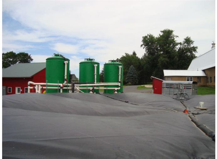
Methane gas flows along the black plastic top of the digester in the foreground. Three scrubbing tanks separate the hydrogen sulfide and water from the methane gas at Barstow's Longview Dairy.
